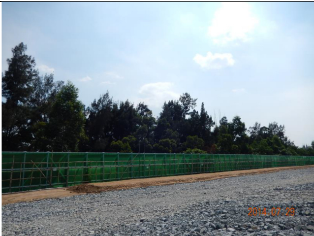
Photo 1: The Construction works have been screened by hoarding (CM2)
