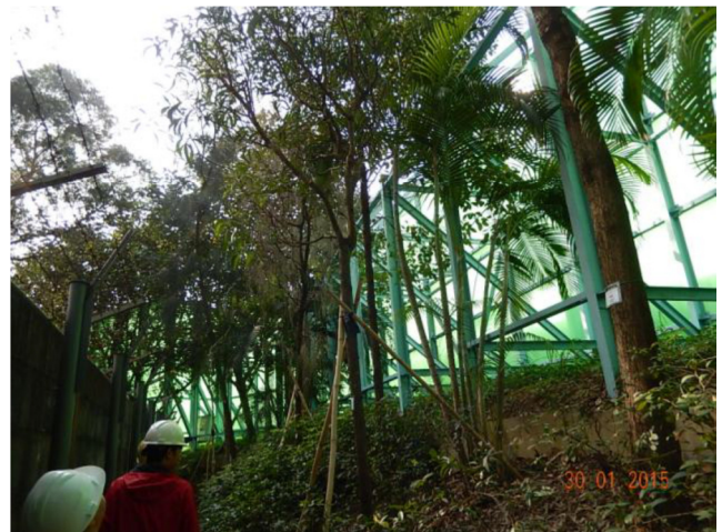
Photo 4: Advance screen planting of noise barrier has been undertaken. (CM6)
