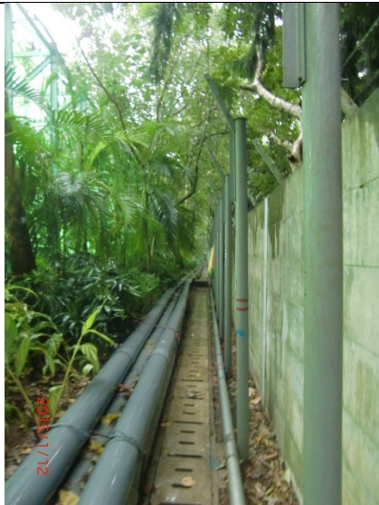
Photo 3: Continuous belt of screen planting along the southern and western boundaries of the site has been completed. (CM6)
