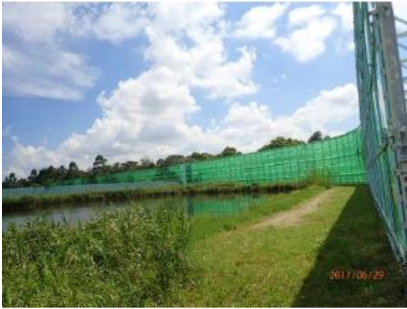
Photo 1: The Construction works have been screened by hoarding / noise barriers. (CM2)
