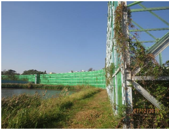
Photo 1: The Construction works have been screened by hoarding / noise barriers. (CM2)
