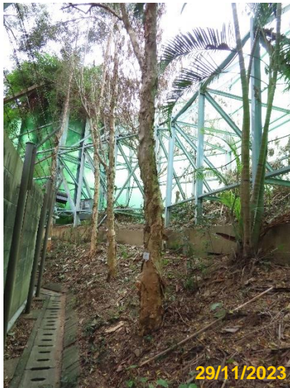
Photo 3: Advance screen planting of noise barrier has been undertaken (CM6, OM2)
