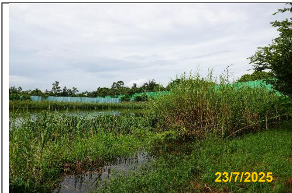
Photo 1: The Construction works have been screened by hoarding / noise barriers. (CM2)
