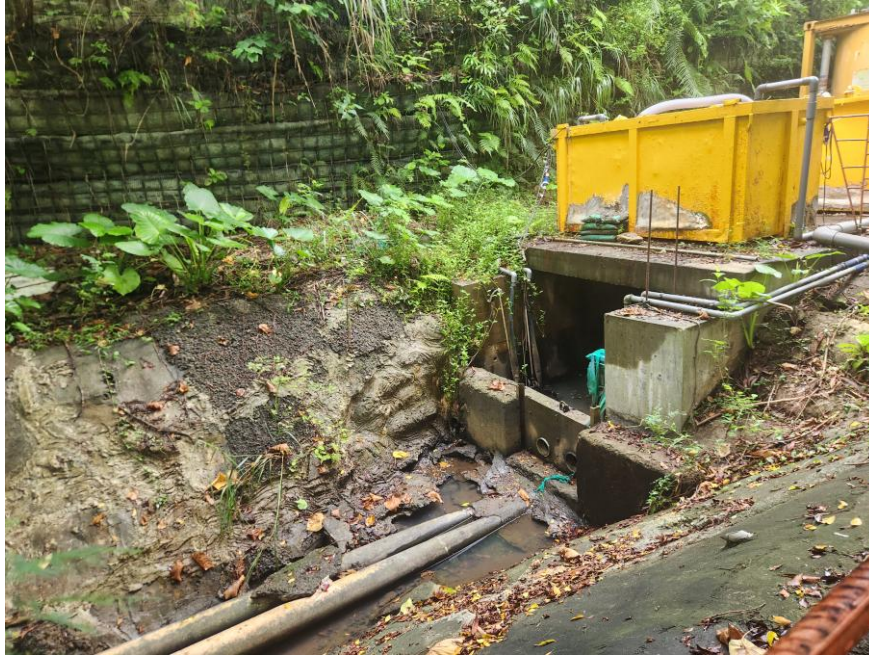
Photo 2 Wastewater treatment facilities (AquaSed, sedimentation tanks) inside the site (near discharge outlet to the northern ditches) on 7 August 2026
