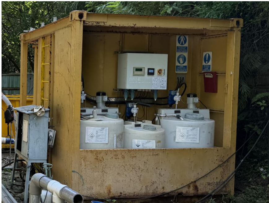
Photo 2 Wastewater treatment facilities (AquaSed, sedimentation tanks) inside the site (near discharge outlet to the northern ditches) on 7 August 2026
